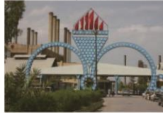
REFINERY Iran 1000 t/h, 40 bar
