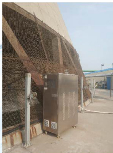
火电厂专用冷却水处理系统 Cooling Water Treatment System for Thermal Power Plants
