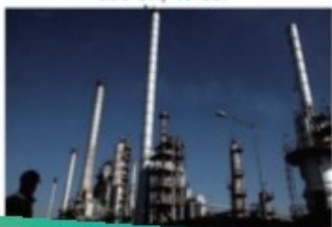
REFINERY Tehran, Iran 800 t/h, 40 bar
