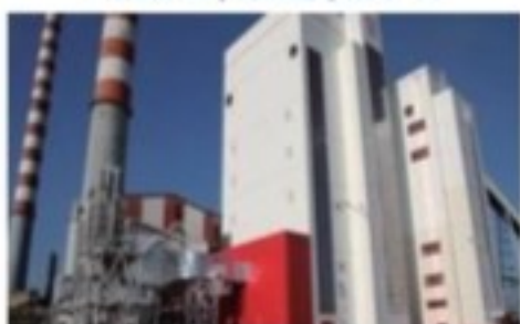
REFINERY Ploiesti, Romania 1 x 23 t/h, 35 bar, 348° C
