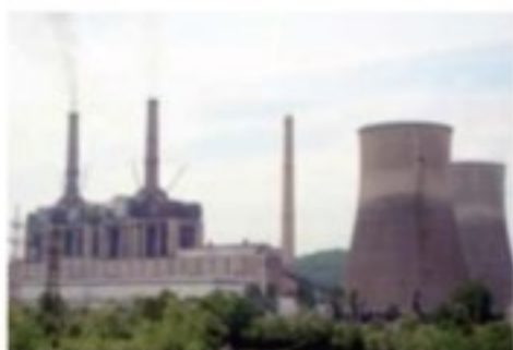
ALUMINIUM REFINERY Tulcea, Romania 2 x 100 t/h, 100 bar, 540° C
